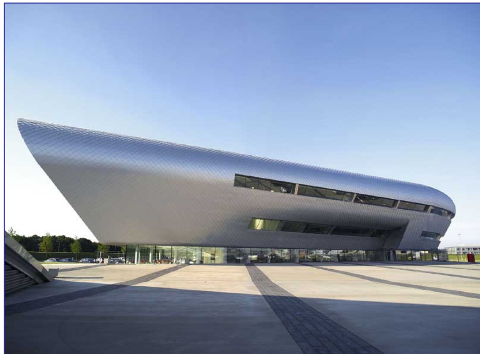
Farnborough Airport Terminal Building
